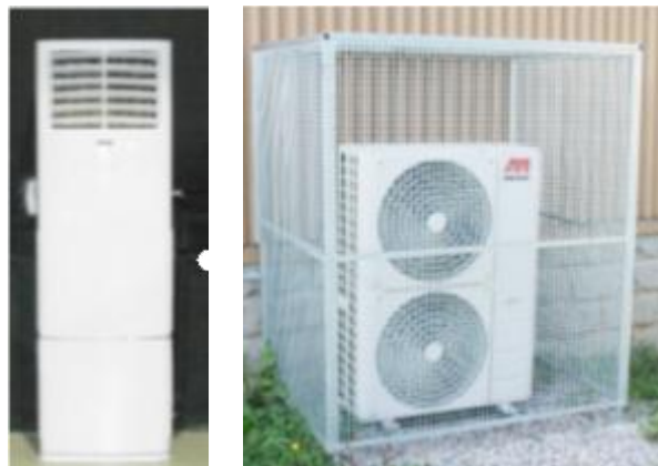
ASHP - Internal & External Components
